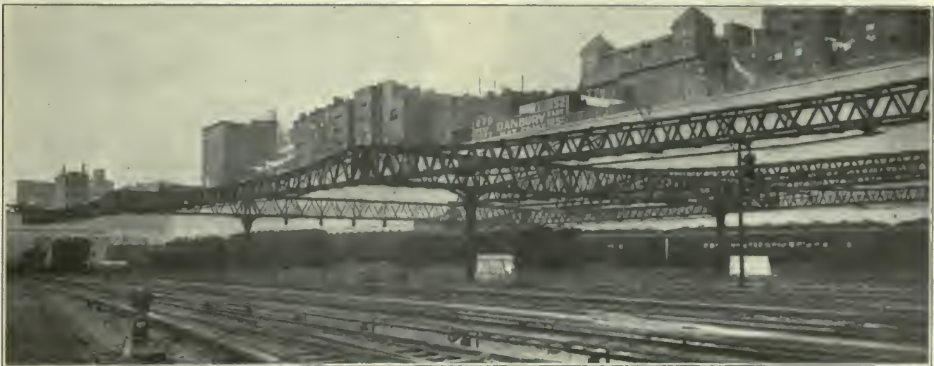
FIG. 510. OVERHEAD THIRD RAIL CONSTRUCTION, TERMINAL AREA, PENNSYLVANIA RAILROAD PASSENGER STATION, NEW YORK CITY
